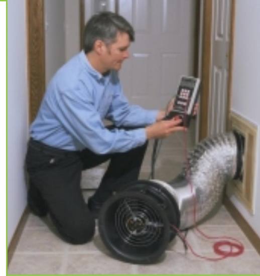
A Weatherization technician conducts a vent test to identify duct leakage.
