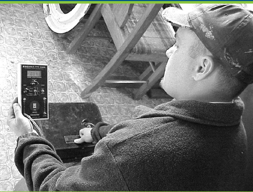
Delaware crews use a digital manometer to identify duct leakage.
