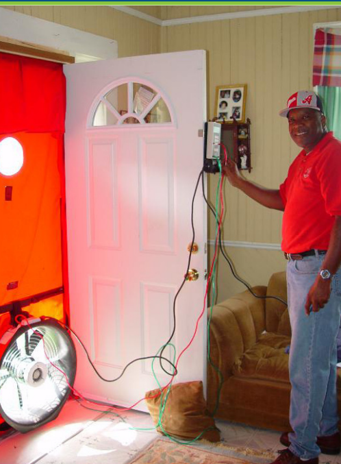
Blower door tests are conducted during the assessment of a weatherization home.
